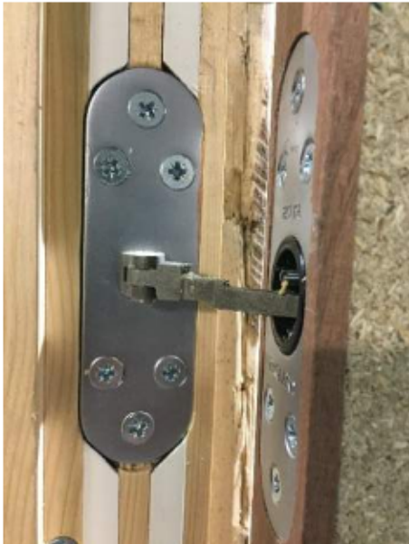
Around concealed closer – both doorsets
